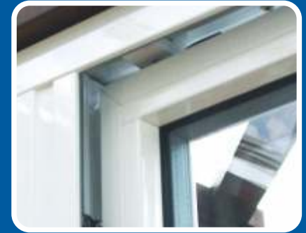
Secure Night Vent Facility
